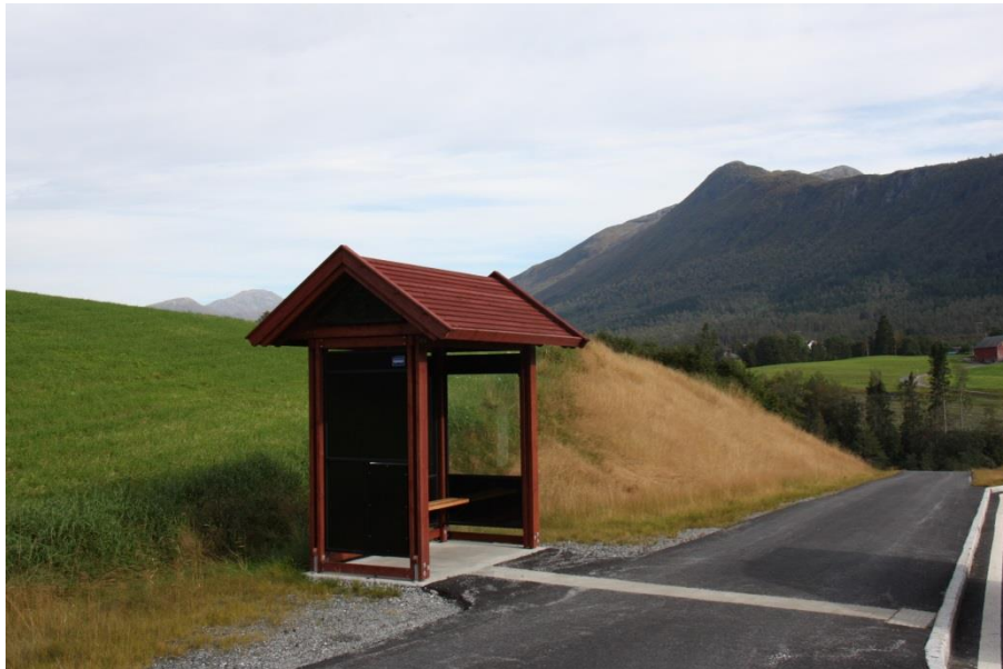
Kvivsvegen, in western Norway. Universally designed bus stop. Step-free access and excellent visual and tactile contrasts. Bench with armrest.
