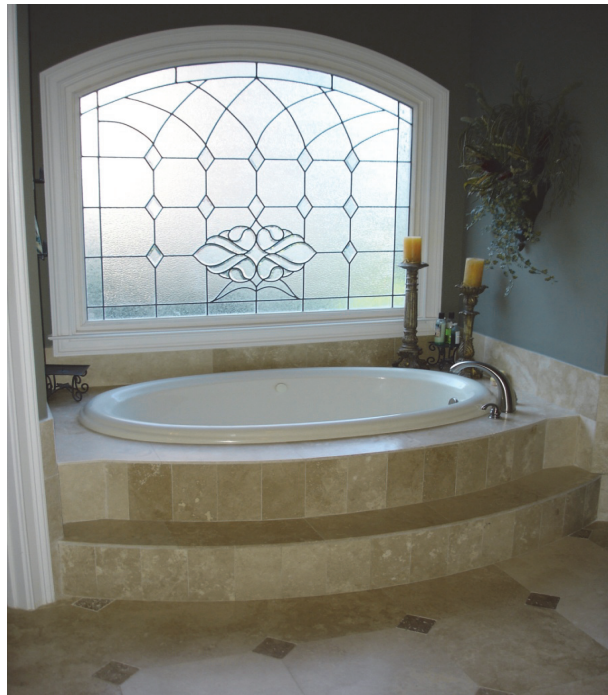
Figure 2. Example of bathtub with potential fall hazard Source: Designs Anew Houston LLC, 2013
